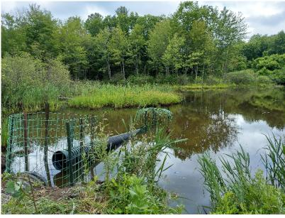
If a beaver site is assessed and determined to be a good candidate for a water flow device, it is important to use proven construction designs, and high-quality materials. Also, be sure to monitor the device, and conduct routine maintenance as needed. It is a rewarding experience when the needs of people and beavers can be met, where their "paths cross" along the varied and diverse waterways of Maine. Ben Nugent, Wildlife Biologist, USDA APHIS Wildlife Services
